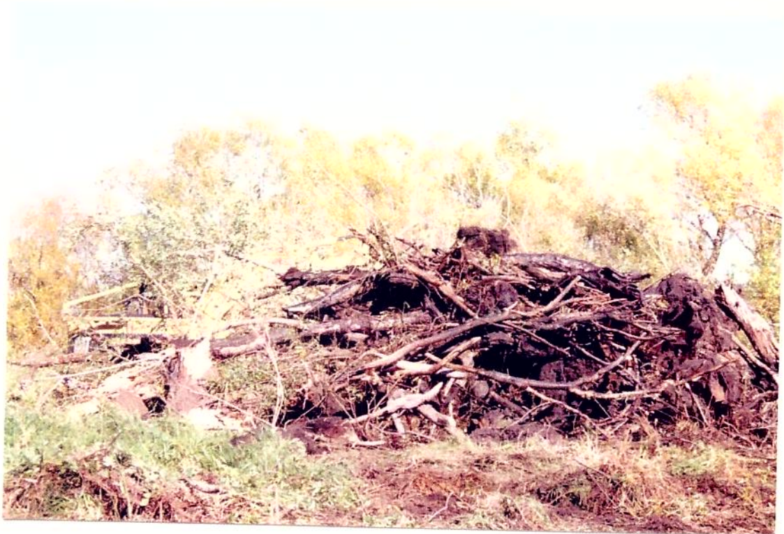
Excavator stacking debris, Eliza Farm, Campania.
