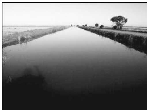
Supply channels are sources of conveyance losses.
