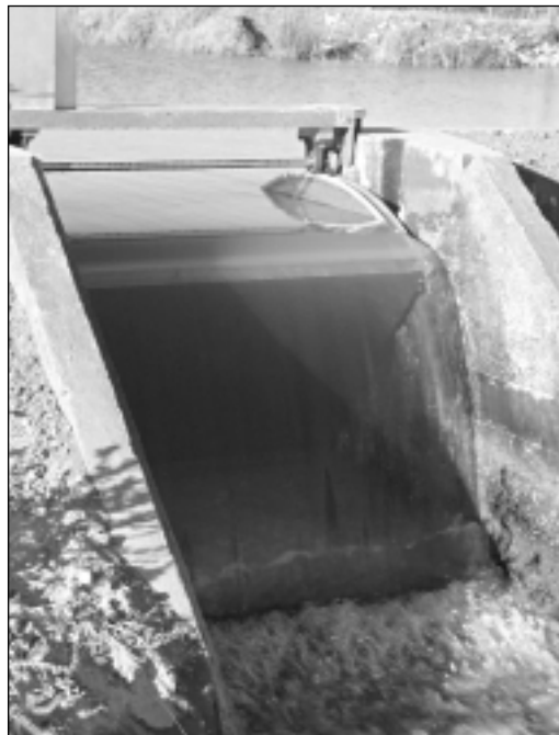
Remote-controlled channel gates allow managers to control and operate the whole channel network remotely and in response to changes in the system.
