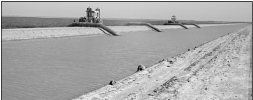
Irrigation with over the bank siphons
