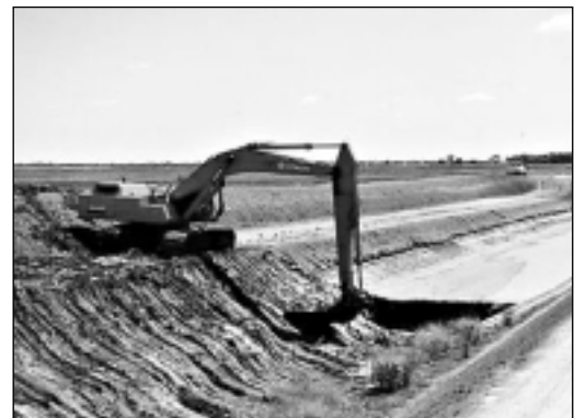
Desilting a channel.
