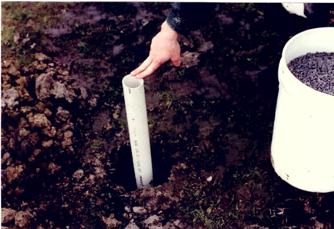
Plate 12. (as in Plate 11) Installation of bore prior to backfilling with gravel and capping with bentonite.
