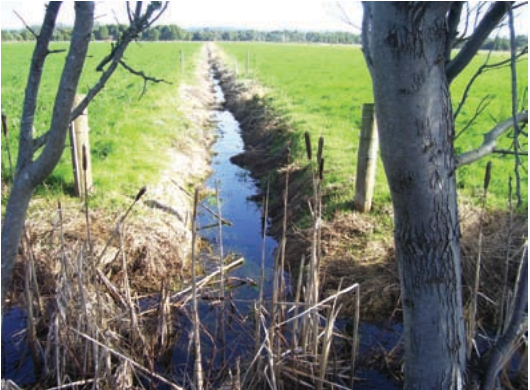
Figure 26. Open arterial ditches lower the water table and remove water from paddocks.
