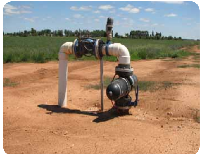
In field secondary filter and control valve
